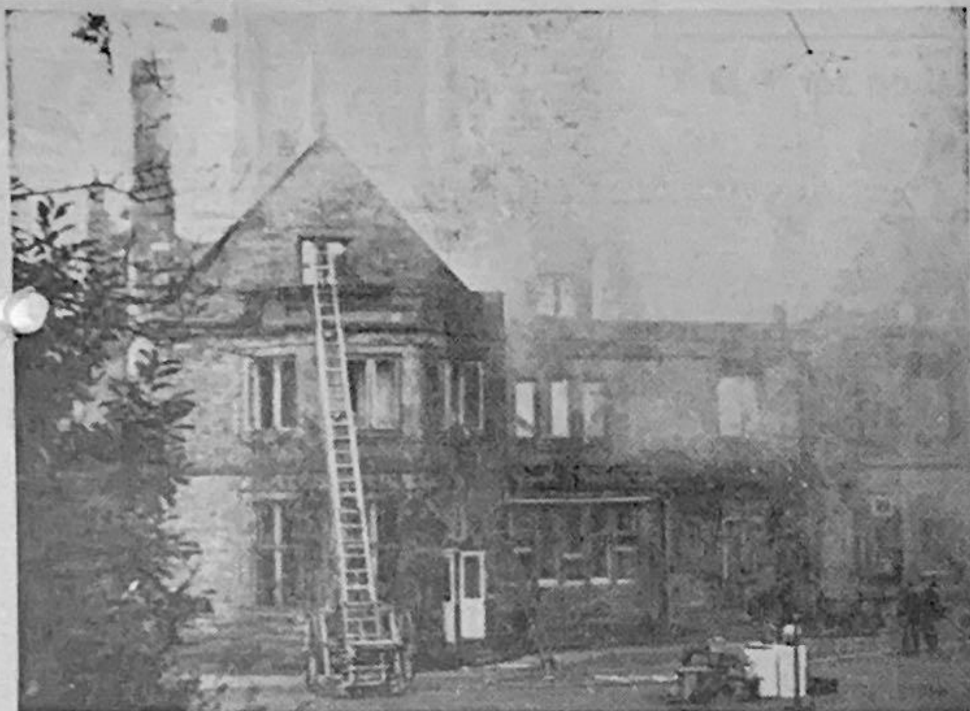
The fire-damaged buildings of Newells Preparatory School, Lower Beeding, where a young Indian boy died as he tried to rescue a school friend.
